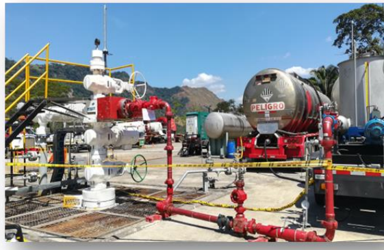
Figure 7. Surface set up for Dispersed Foam Deployment at well location
